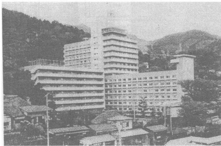
Figure 20. General view of retrofitted building with seismic isolator at mid-story 1)
